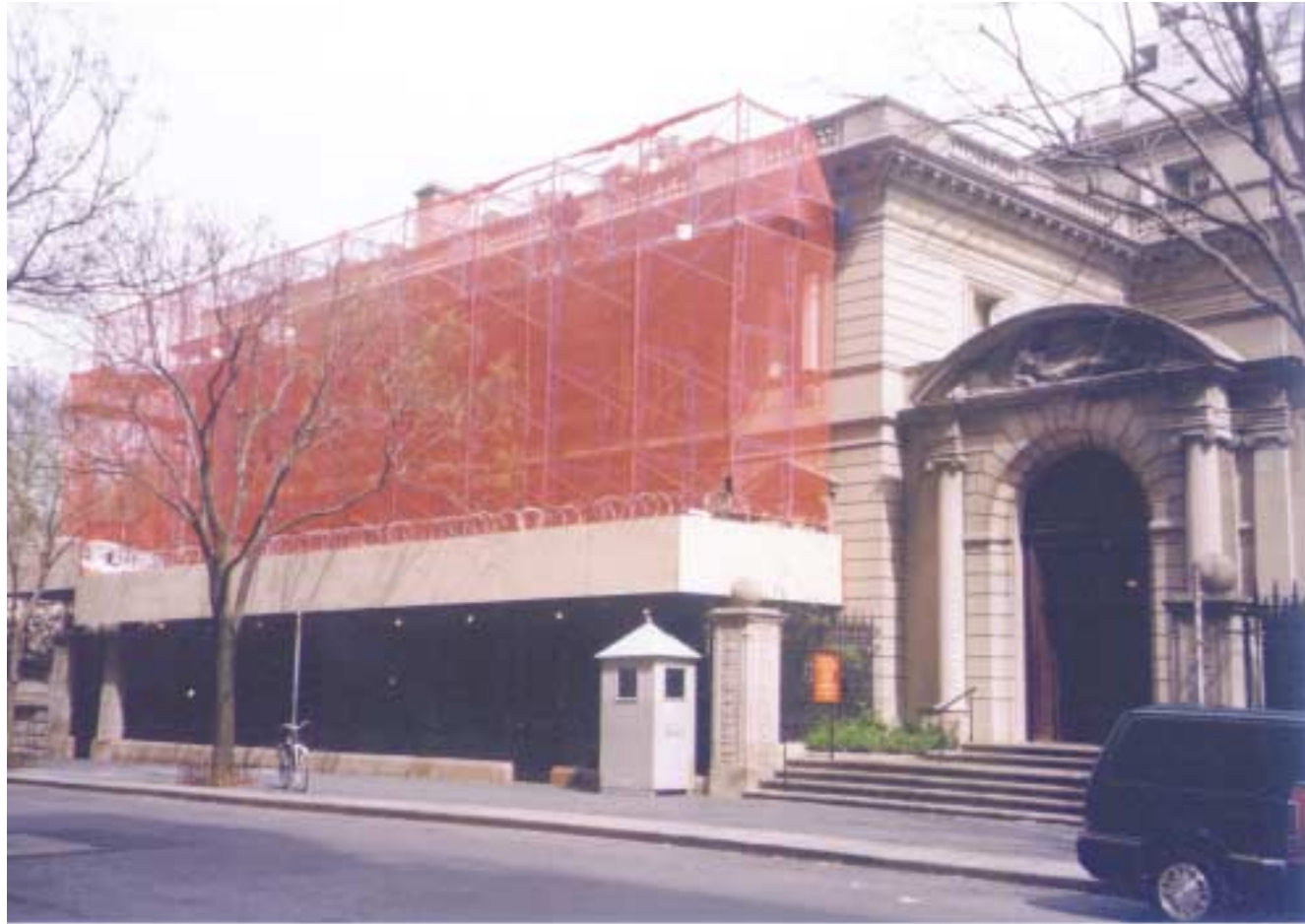
Last spring, scaffolding went up while stonework restoration was completed on the building's entire façade. Further work on the walls surrounding the Fifth Avenue and Seventieth Street gardens will continue through summer 2001.
